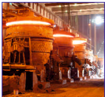
IRON & STEEL PLANT
